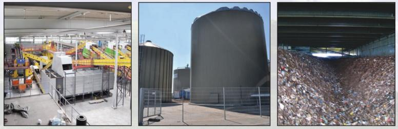
ECOCOM offers the most modern and complex solution in order to provide an environmentally safe waste treatment. Mechanical biological waste treatment plants are a combination of mechanical sorting and a 2-stage dry or wet anaerobic digestion (fermentation). Mechanical sorting is used for separating the waste into several streams to enable specific recycling and disposal. In this stage the fine organic fraction will be sorted out for the further anaerobic digestion (fermentation).
